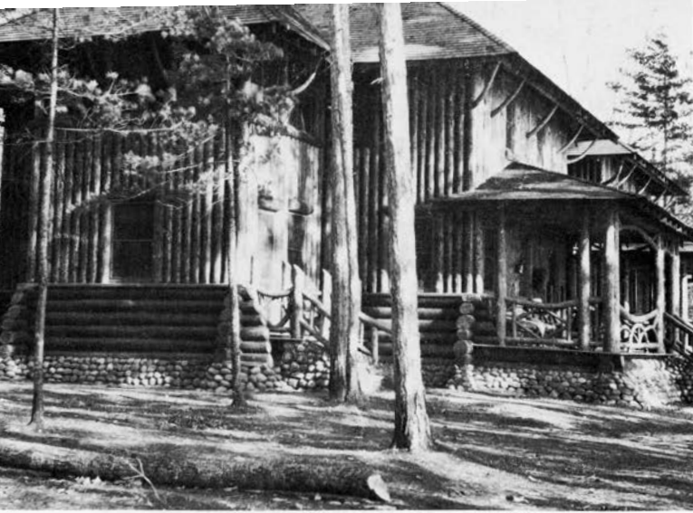
Forestry headquarters, Trout Lake. The near extension was the office for Assistant State Forester Moody, and included the switchboard for the 4 lines to the lookout towers.
