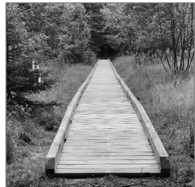
A new boardwalk carries students over the wetlands to help preserve the ecosystem.
