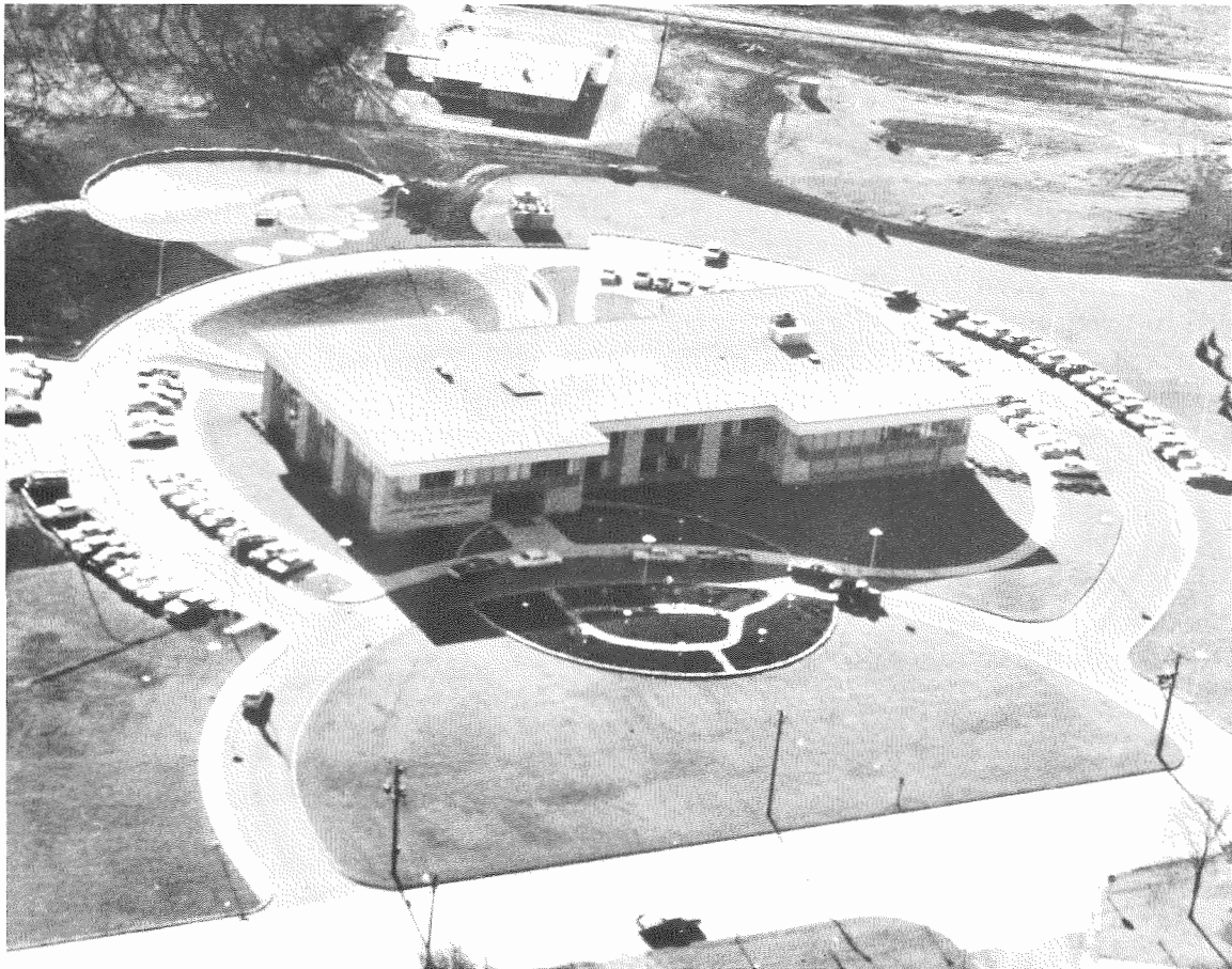
Completed home office in the shape of a bold faced "H", 1963.
