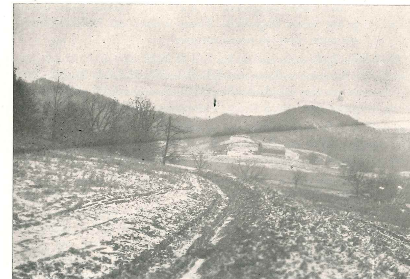
Diversion terrace on the Orville Jost farm, fall of 1922.
