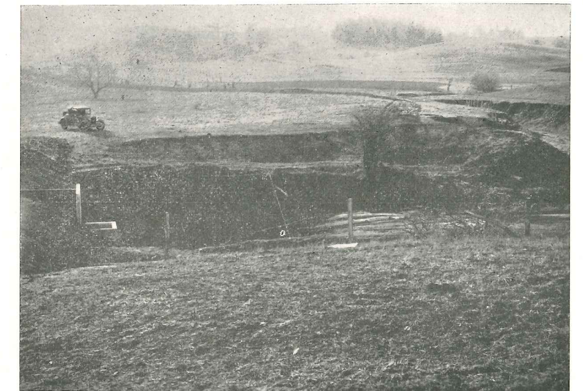
CCC drop inlet dam. Earth dam is below concrete inlet at extreme left. Gully above dam will eventually fill with soil lost from the watershed even if good erosion control practices are used.
